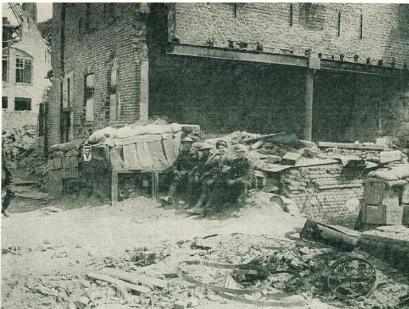
Another YMCA canteen, this time a "dug out" under ruined buildings in the shattered town of Ypres in June 1917.
